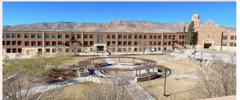
Austin High School Courtyard Renovation
