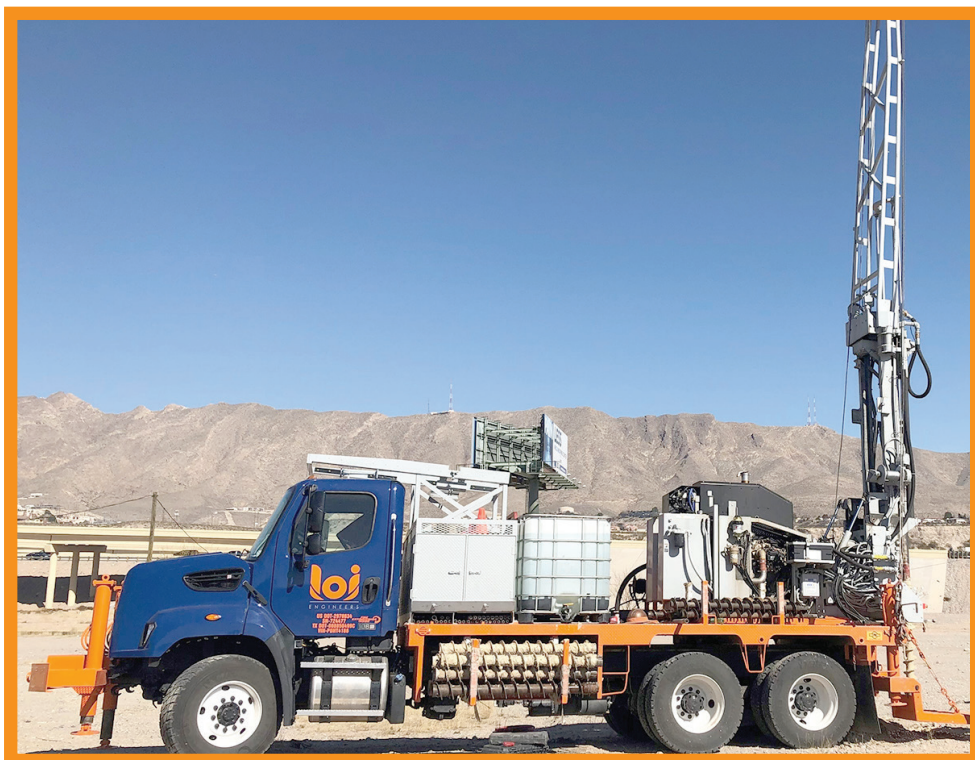
One of our drilling rigs at EPWater’s Hickerson WWTP (February 2023) site.
